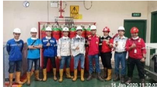
Fire Alarm & Clean Agen System CPBL PT Adaro Indonesia-Kelanis
