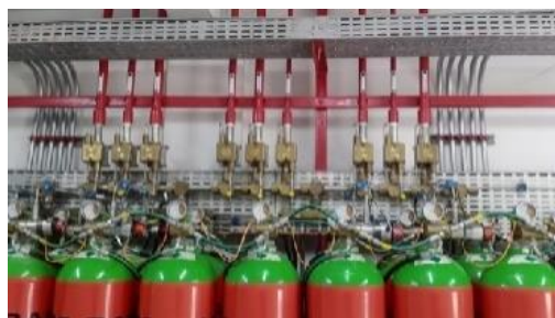
Inergen Fire Suppression System PT Adhi Karya (Persero) Tbk Kereta Api Ringan (Light Rail Transit)
