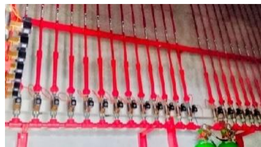
Inergen dan Co2 Fire Suppression System PT. Multi Artha Pratama Gold Coast PIK (RS. Buddha Tzu Chi)
