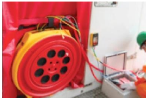
Room Integrity Test Gas Turbine BP Tangguh
